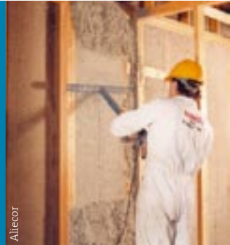
Application de fibres isolantes
